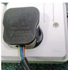
Ensure no taped or inappropriate joints.
